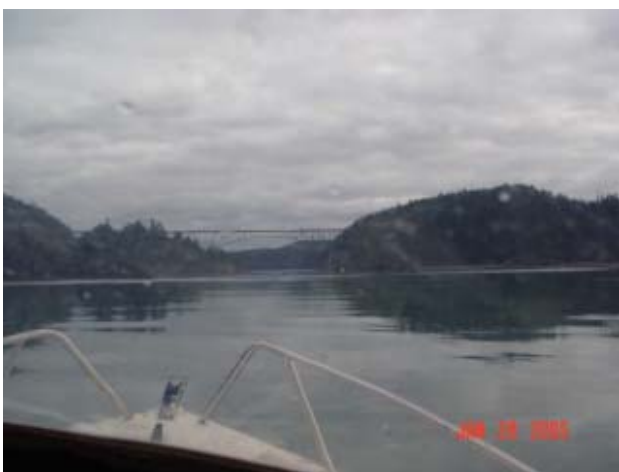
The bridge over Deception Pass joins Fidalgo and Whidbey Islands.
